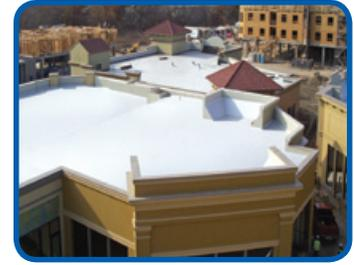
**SOPRASTAR uses a patented tri-laminate synthetic film that adheres on top of the SBS membrane. Competing products use a factory-applied coating or synthetic chips fused to a granular surface.**
